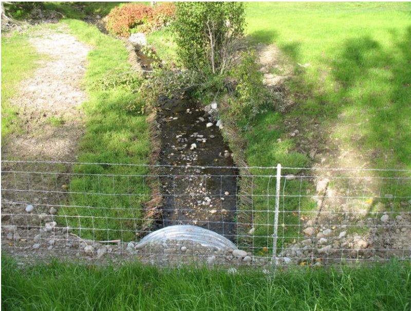
Sunrise Road: New, larger and embedded culvert.
