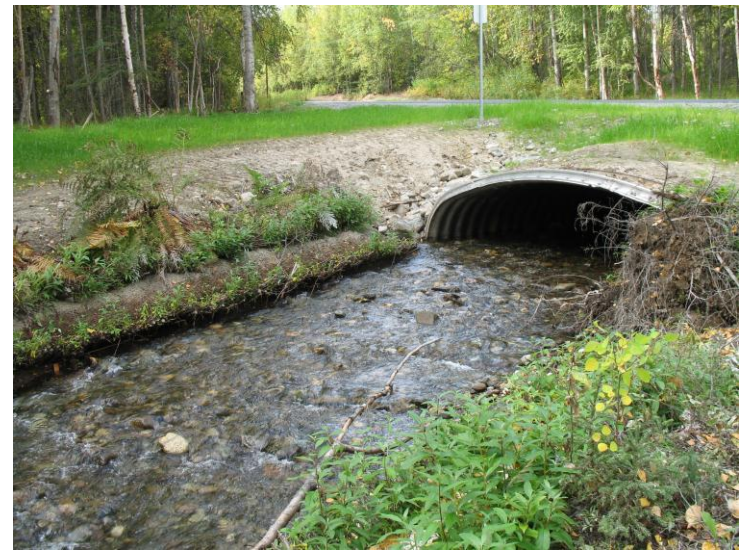
Coyote Creek new 19 foot box culvert.
